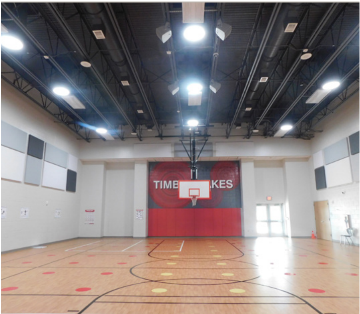
TOC Open ceiling
