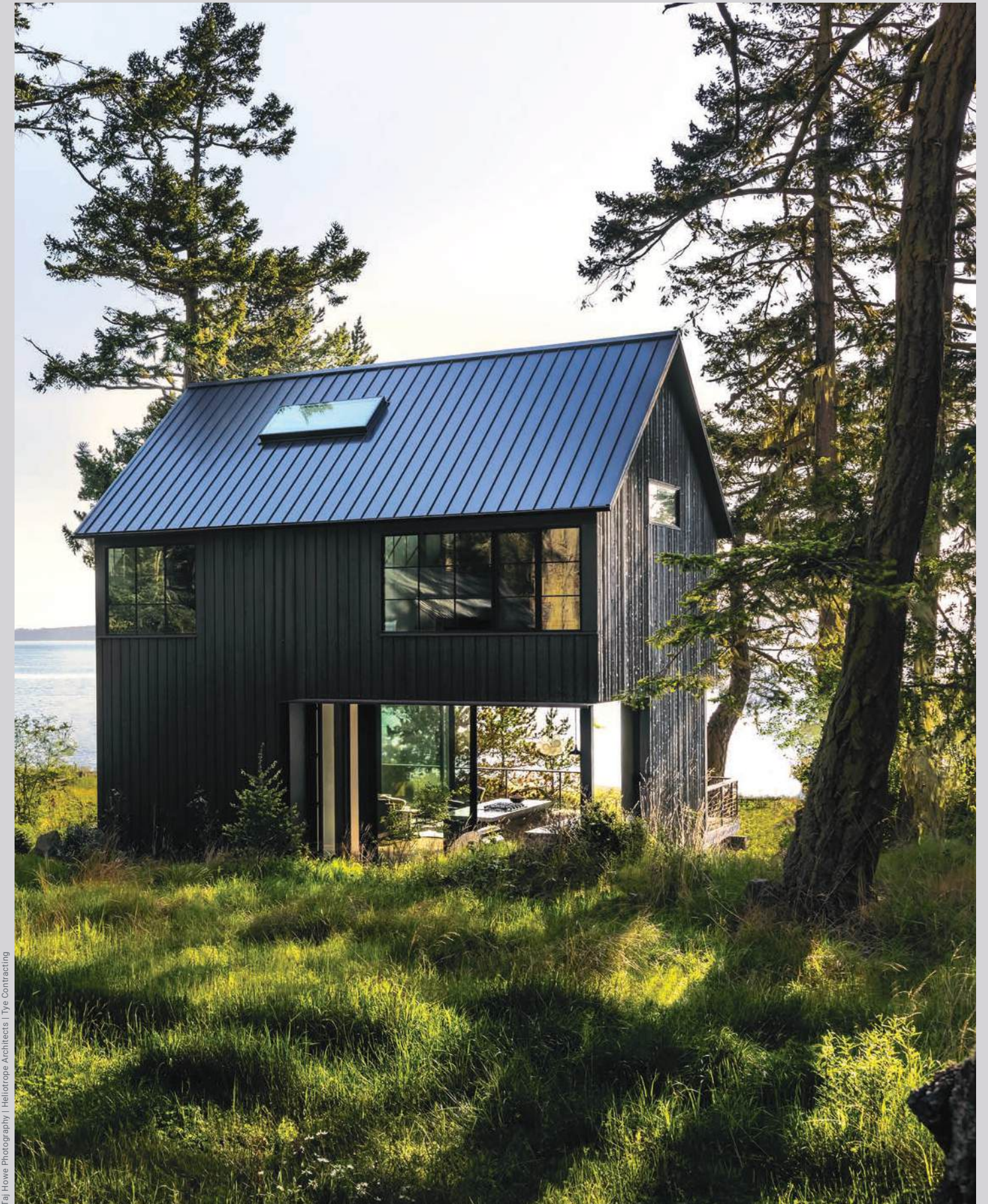
Taj Howe Photography | Heliotrope Architects | Tye Contracting
