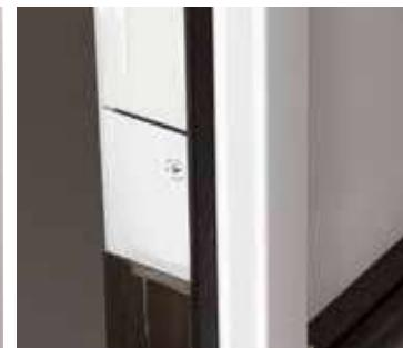
Astragal bolt penetrates threshold allowing boot to seal, creating a better barrier against the elements
