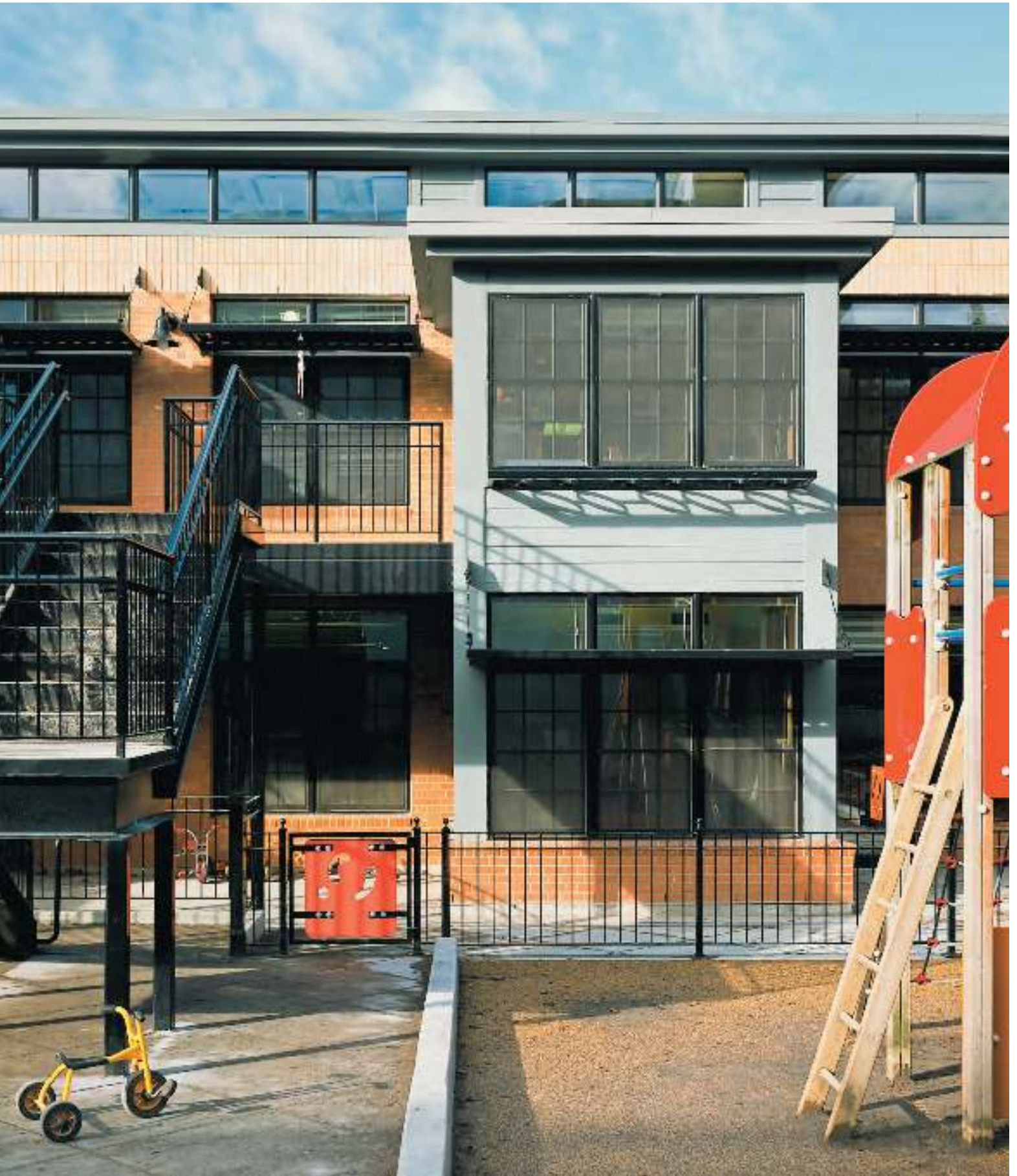
Helen Gordon Child Development Center Portland, OR GBD Architects E-Series Windows and Doors
